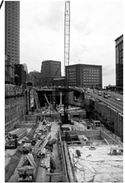
July 2003, Fort Point Big Dig Construction
