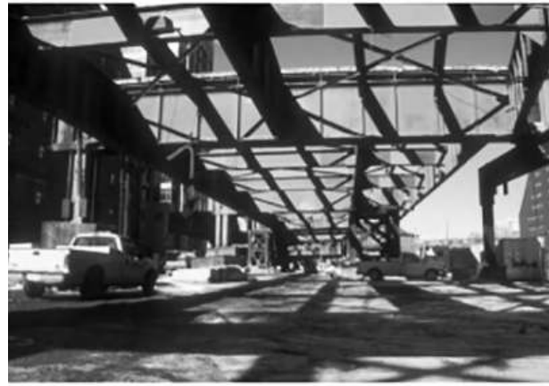
2004, Partially-demolished underpinnings of Elevated Highway
