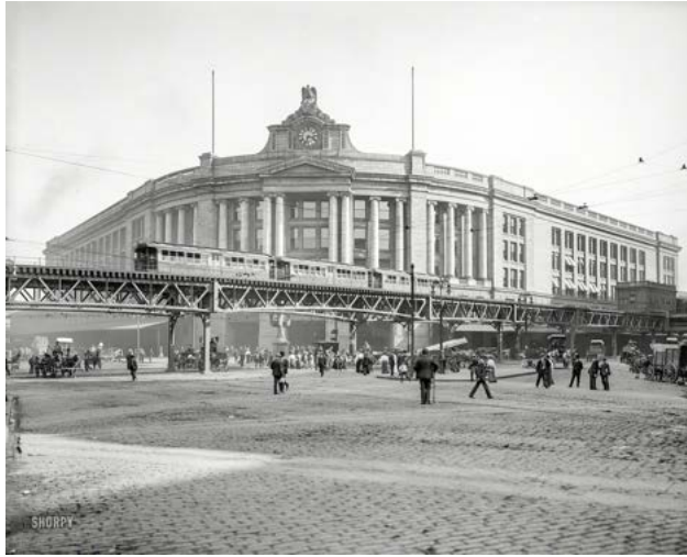
1905, South Station & Elevated RR
