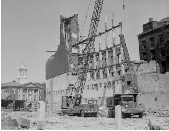
1952, Demo near entract to East Boston Tunnel
